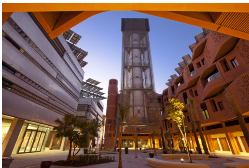
Fig 13: Masdar institute central courtyard and the wind tower. (Copyrights: Nigel Young/ Foster+Partners)
